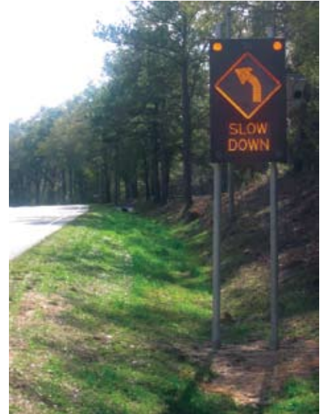
Florida state DOT VATCS install District 3 Tallahassee
