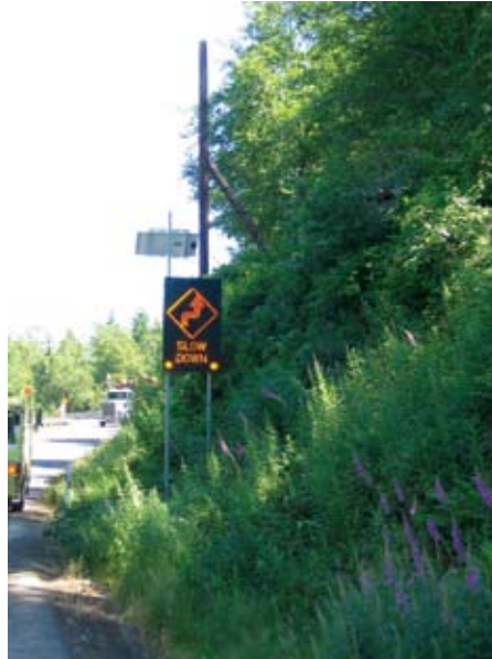
Washington State DOT VATCS Install Olympic Region
